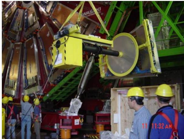
**Fig. 11.** Installation of a muon chamber on the iron disc of the magnet return yoke
