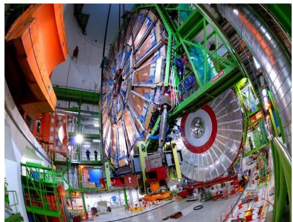
**Fig. 12.** The lowering down of one iron disc with muon chambers in the underground hall
